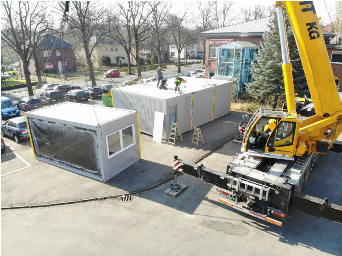
Picture 1: Assembly office container
